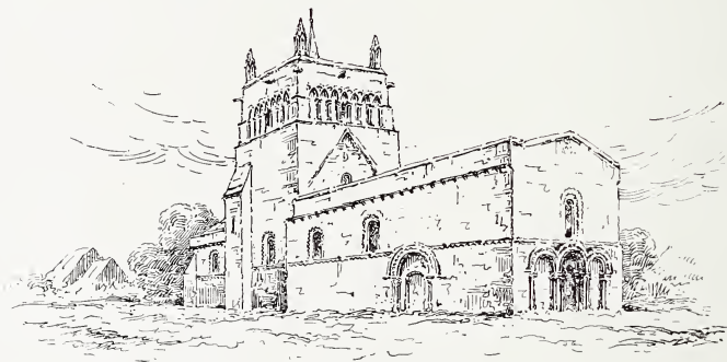
51. STEWKLEY FROM THE NORTH-WEST
